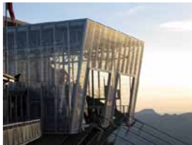
Stanserhorn Bahn, CH – 840m 2 single layer ETFE
