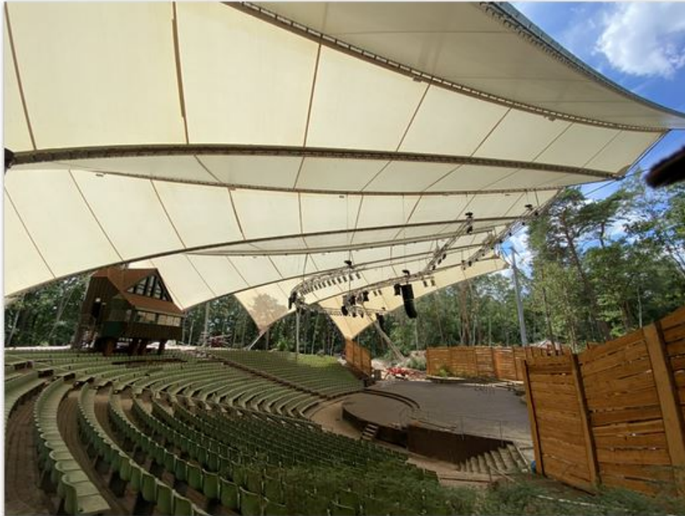
The roof construction combines aesthetics and functionality and offers protection from rain and sun. Picture: Temme//Obermeier
